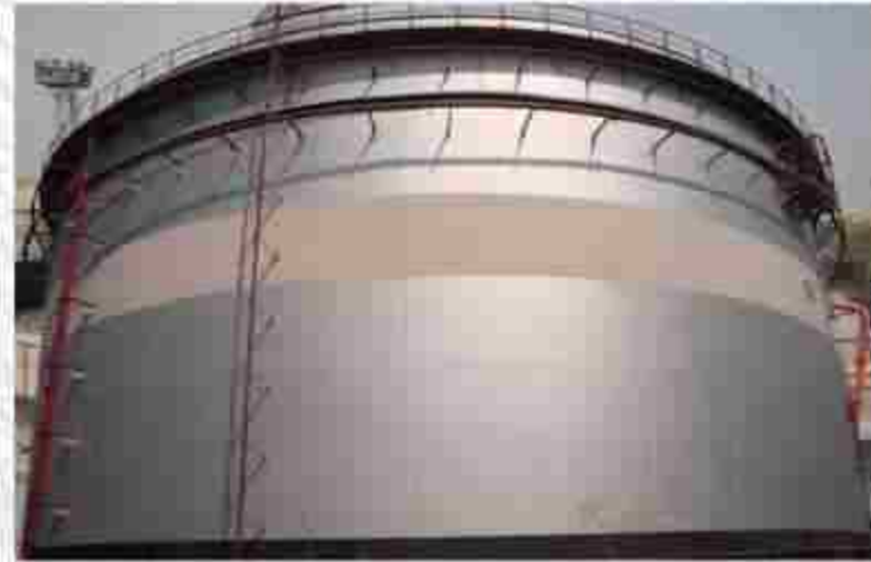
Floating Roof Tanks
