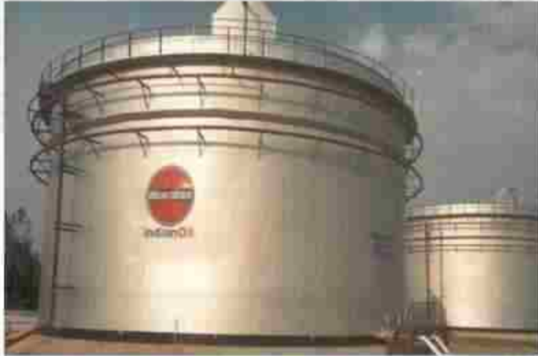
Cone / Dome Roof Tanks
