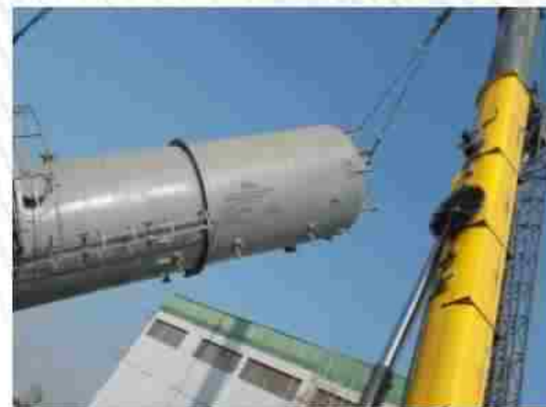
Fabrication & Erection of Equipments
